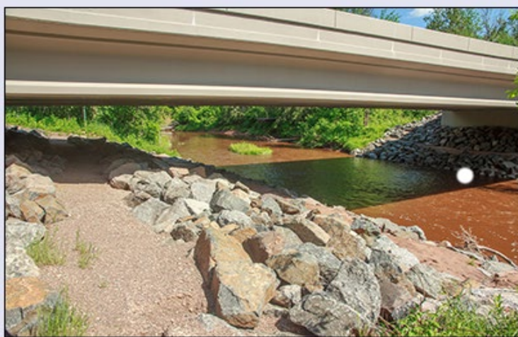
To help deer and other wildlife stay off the roadways, MnDOT uses gravel "passage benches" on most of its river bridge projects. The passage bench is incorporated into bridge riprap and serves to mimic game trails. Wildlife can pass beneath bridges uninterrupted as they travel along the streambank. Photo by Peter Leete
