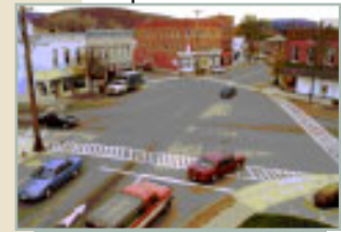
Hanover Square was a five-legged intersection with no clear organization or priorities for vehicle movements.
