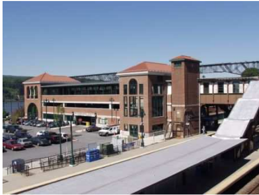
Renovated Metro-North Station Poughkeepsie-Dutchess County Transportation Council
